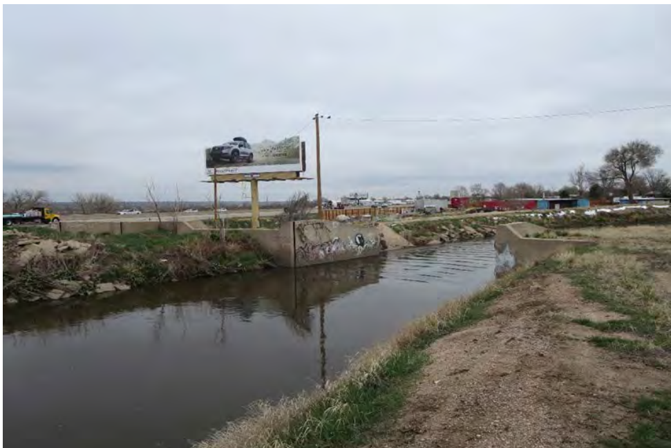
Figure 34. The O'Brian/Burlington Bifurcation site (Feature 1): concrete abutments and diversion box (on left); view to northwest
